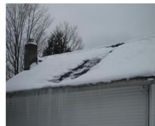
But snow melt patterns can also indicate a problem of too much
