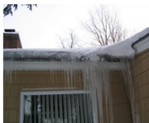
Big icicles themselves, like those shown here, are obvious signs that you're at risk.
