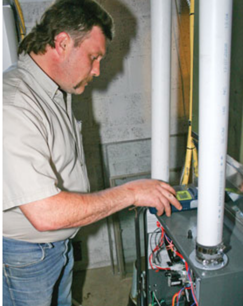
Figure 7. The technician verifies the correct operation of a new furnace and water heater (left) and documents the safety of the new kitchen range (below left). A final blower-door test (below) indicates the increase in house airtightness, from 3,600 CFM-50 to just over 1,900 CFM-50.
