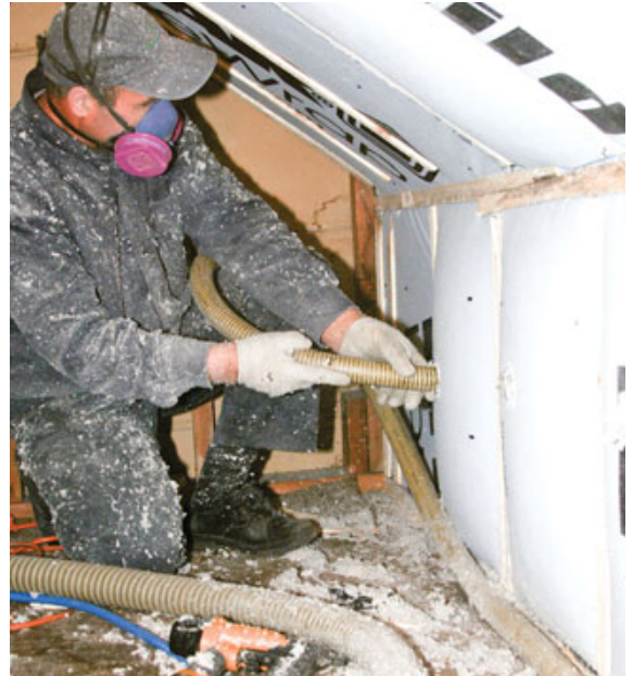
Figure 4. Here, a crew has applied housewrap to the inside face of a knee wall and low roof and is dense-blowing cellulose into the wall cavities (right) and the short sloped section of ceiling (above).
