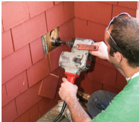
Figure 5. A GreenHomes wall-insulation crew carefully cuts off wood shingle siding to expose the sheathing (far left), then drills holes for the insulation blower hose (left). After blowing in the cellulose (below left), they seal the holes in the sheathing with closed-cell expanding foam (below), then carefully re nail the shingles.
