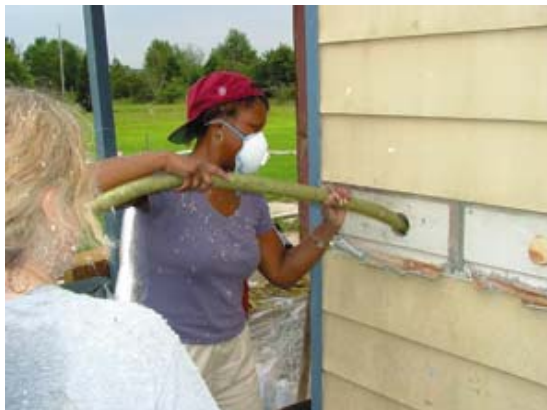
Dense-packing insulation in the side walls can boost a home's energy-efficiency.
