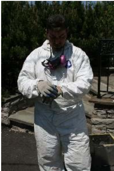
A GreenHomes crew member suits up for attic insulation work.
